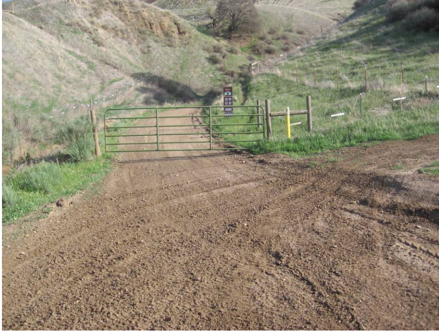
Figure 7. Example of stable conditions. Recent vehicular activity in the foreground show minimal signs of rutting.
