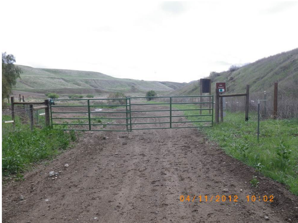
BMP 202-Hills Access Gate
