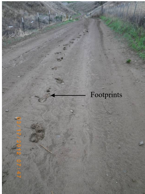
Figure 5. Example of unstable site conditions. The impression of the footprints suggest the site is not dry enough to reopen.
